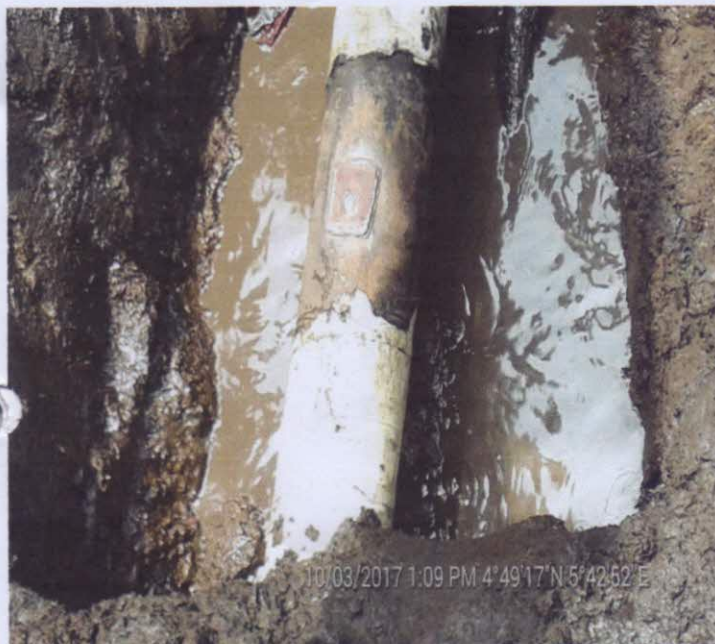
C: PATCH PLATING OF LEAK POINT
