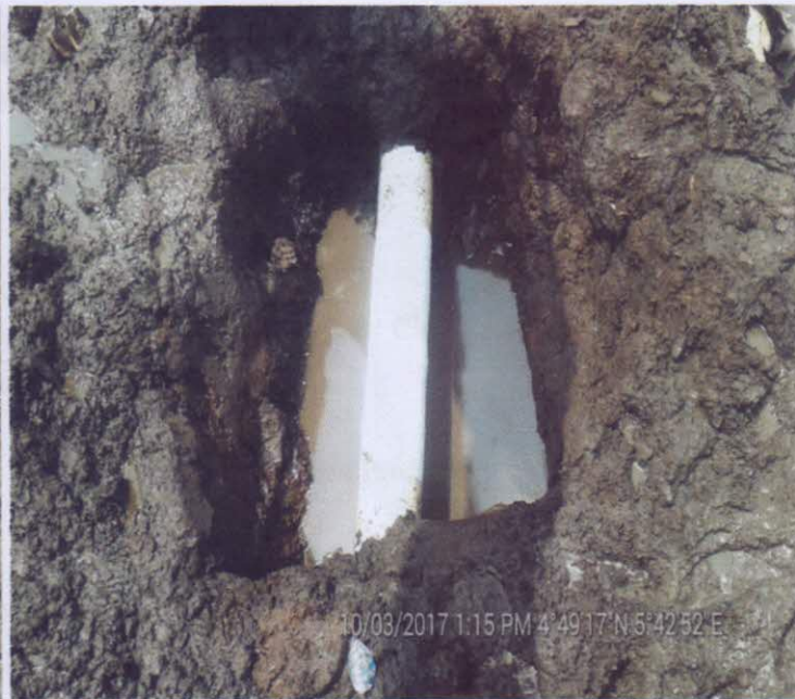
D: WRAPPING OF REPAIRED POINT
